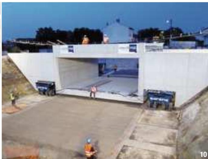
9- Preparation of the bottom of cut for skidding.
