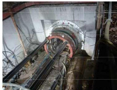
Figure 9. Jacking pit, jacking phase
