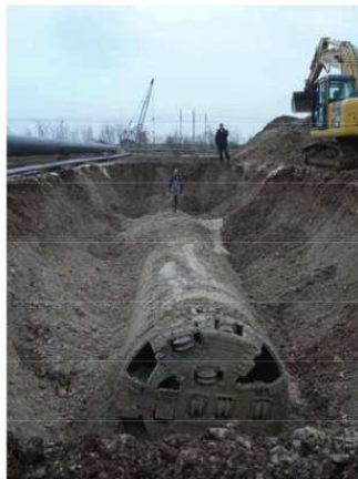
Figure 8. Recovery of the drilling head
