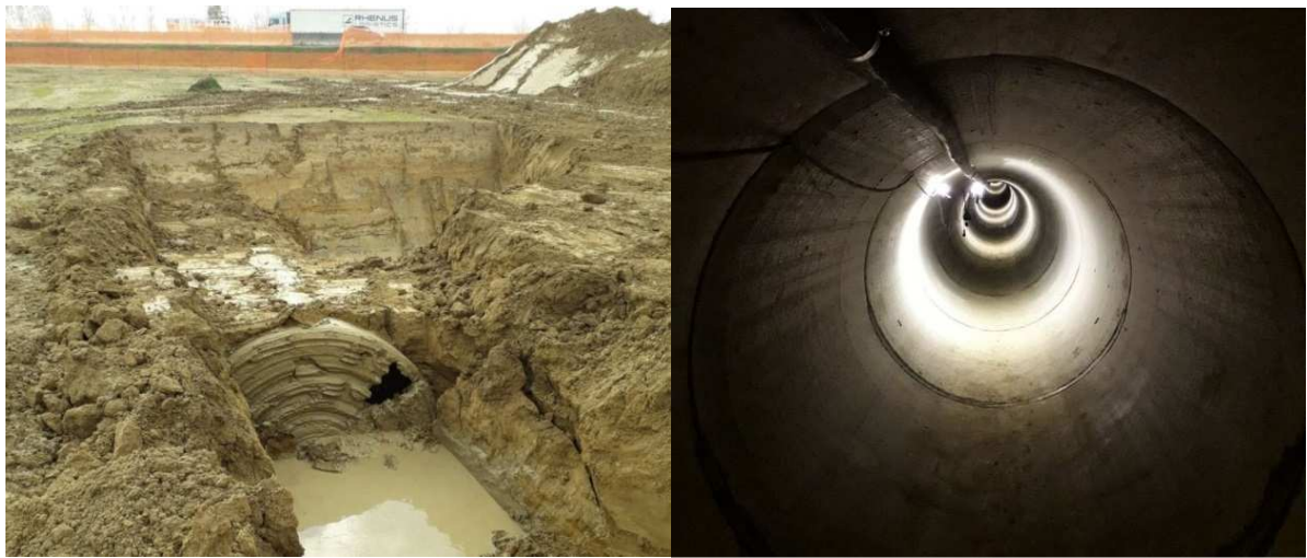
Figure 4. The cutter at the end of the drilling – Figure 5. Alignment of ashlars in the microtunnel
