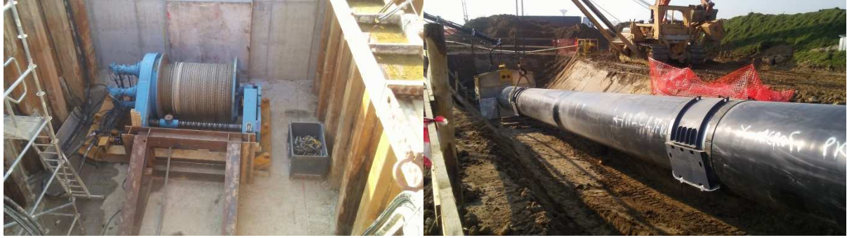
Figure 8. Winch in position – Figure 9. Section of the pipe during the installation phase
