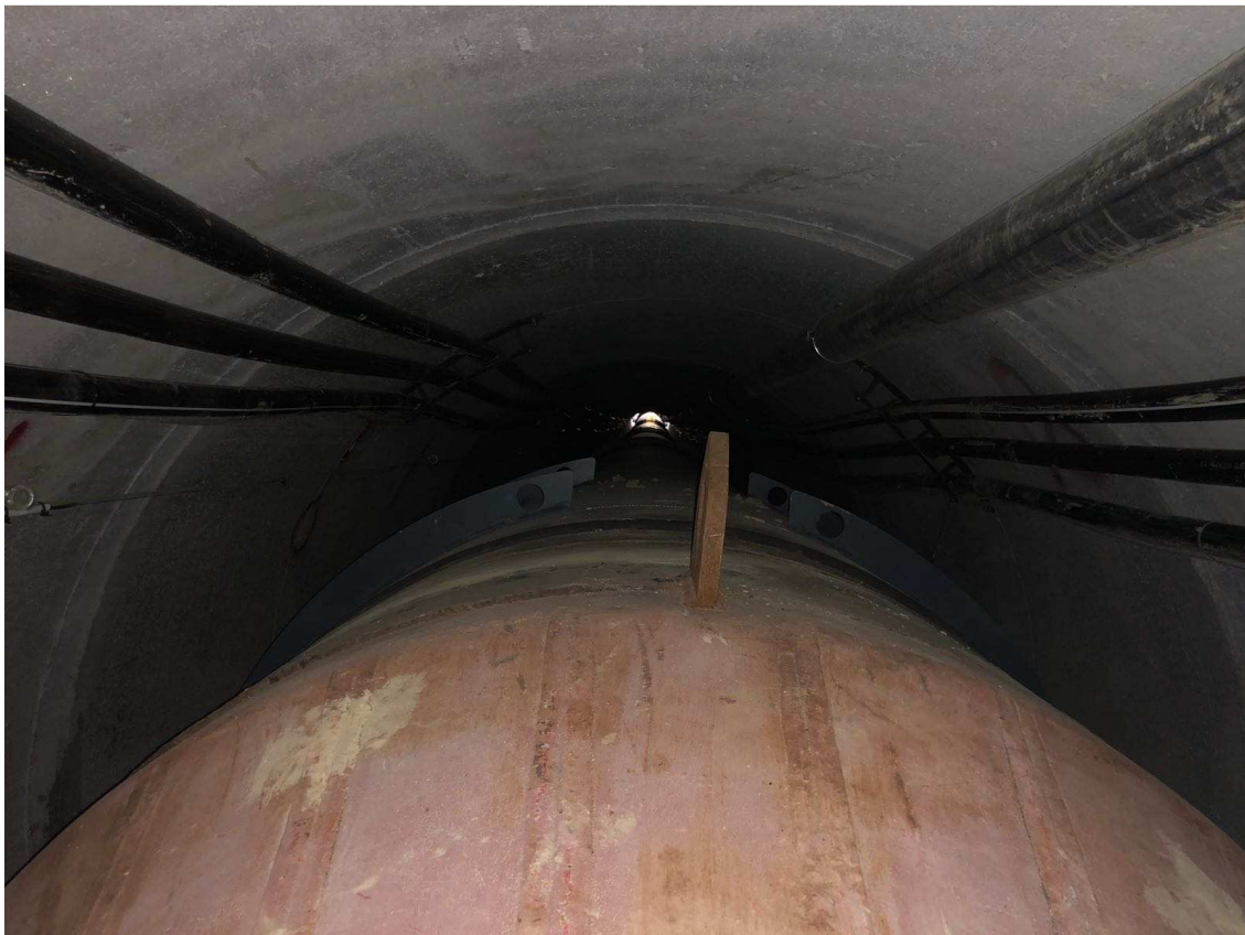
Figure 15. Aligning the pipeline in the microtunnel
