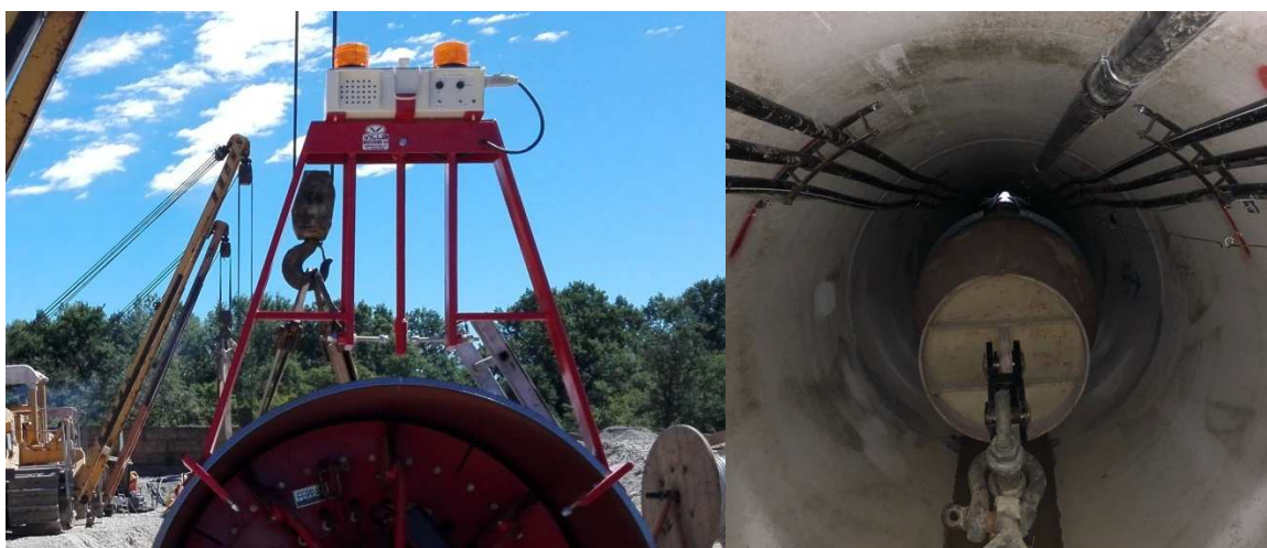
Figure 12. Pendulum for verticality control - Figure 13. Launching head inside the microtunnel
