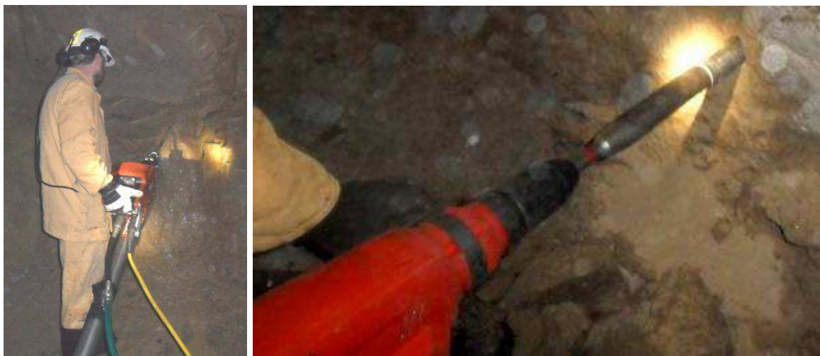
Fig.34. Drilling the holes and fixing the HDA-P bolts
