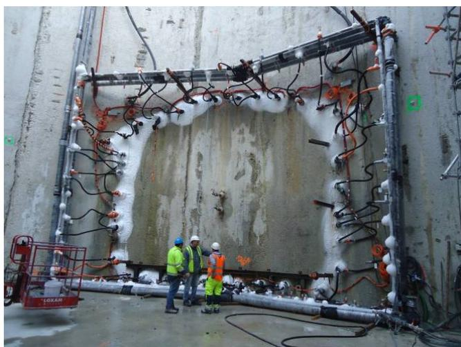
Fig. 8 Freezing phase by Liquid Nitrogen (direct method)
