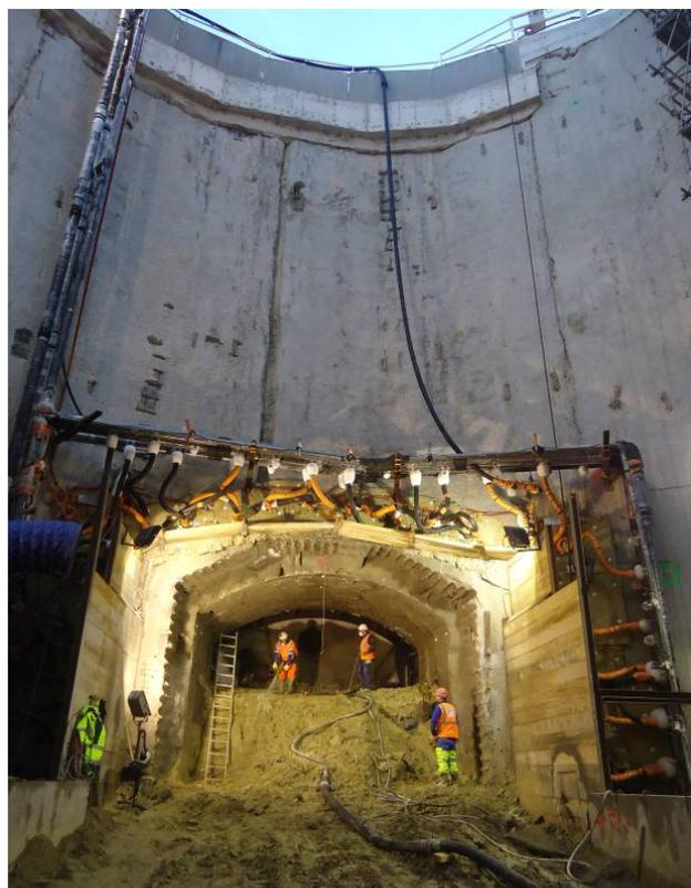
Fig. 9 Passenger Interchange Tunnel excavation front with AGF maintenance ongoing
