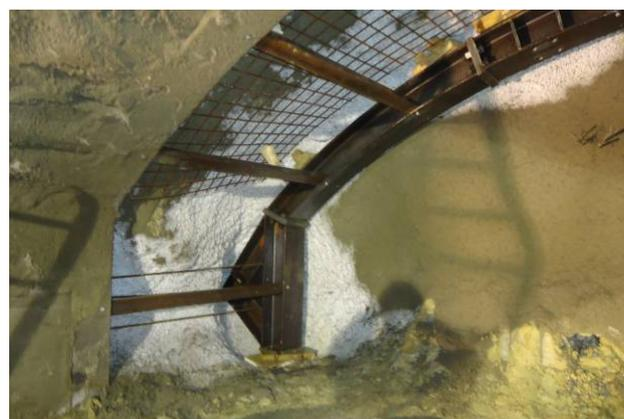
Fig. 10 AGF showing the frozen ground behind the steel sets in place (temporary support)
