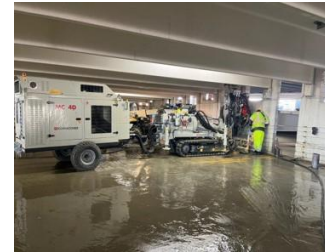
Springfield Parking Garage
