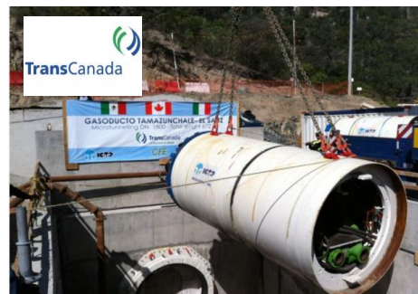
Gasduct Ixmiuilpan (Mx)
